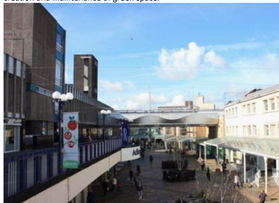
Figure 26: The Merseyway Shopping Centre is a notable challenge however the buildings are highly suited for adaption to hold climbing and rambling vegetation which would have a strong visual impact.
