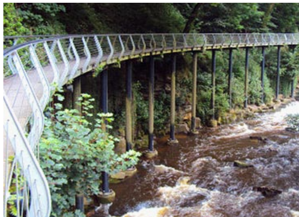
Figure 31: Torrs Millennium Walkway at New Mills.
