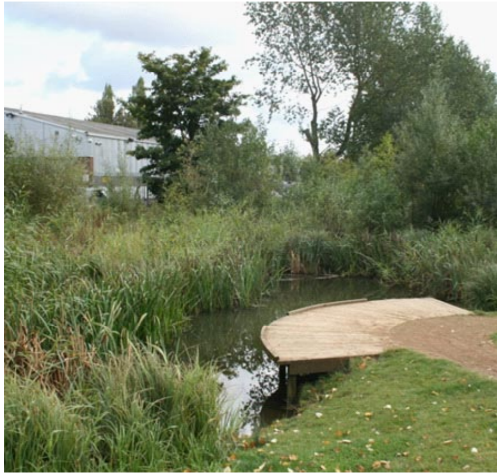
Figure 21 (above): Surface water management with public access providing surface water drainage for a garage franchise.
