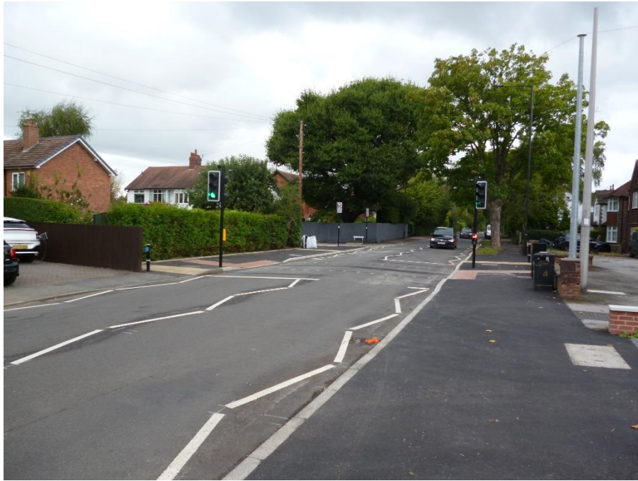
Image 5: Touca Crossing upgrade on Bramhall Lane.
