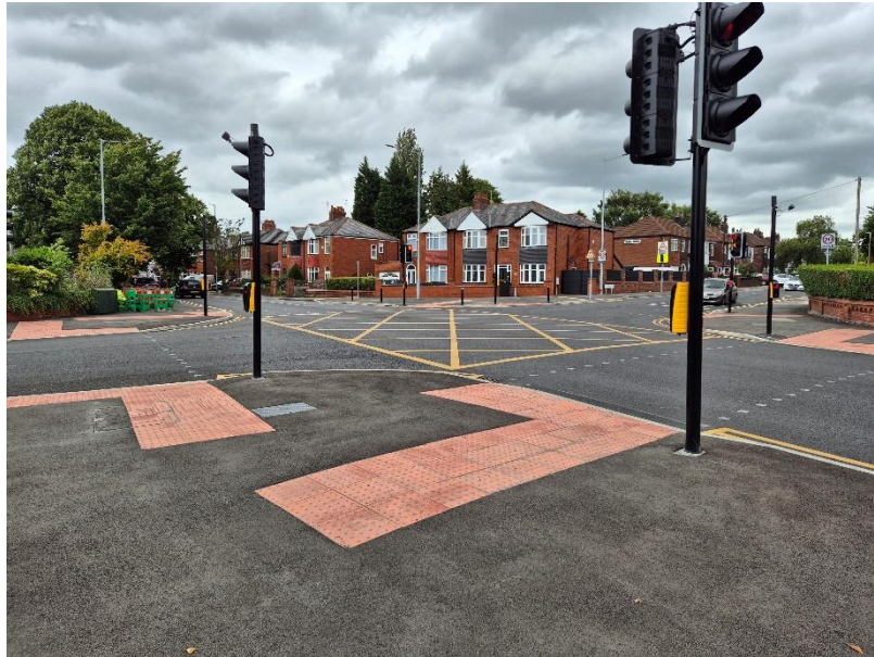
Image 2: New Toucan crossing on Broadstone Hall Rd
