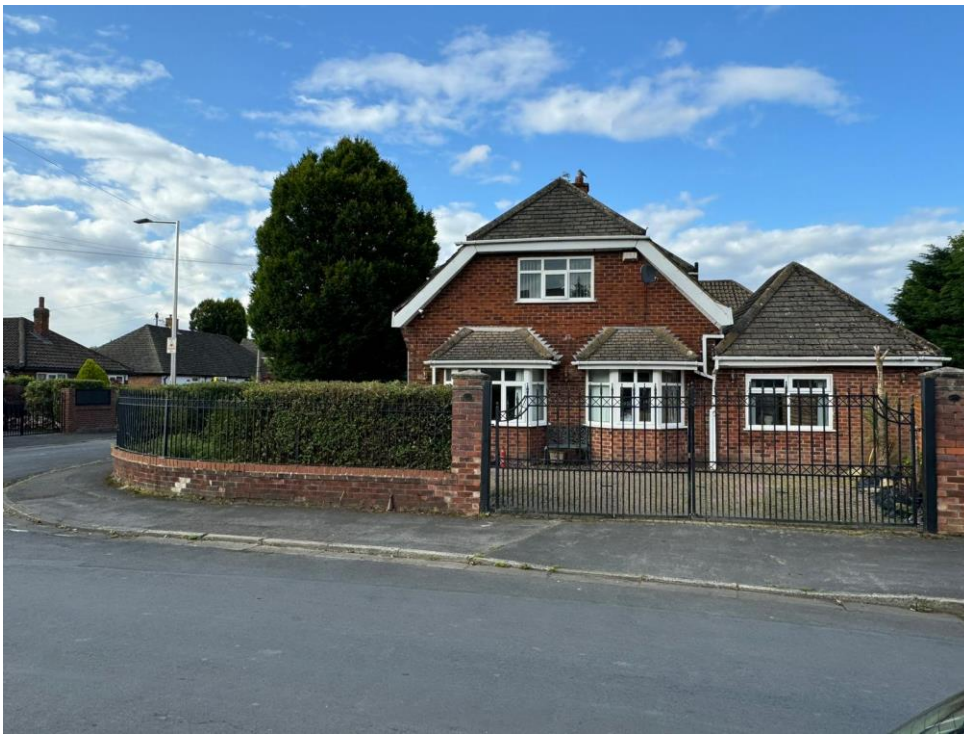
2. Side view from Greenway Road.
