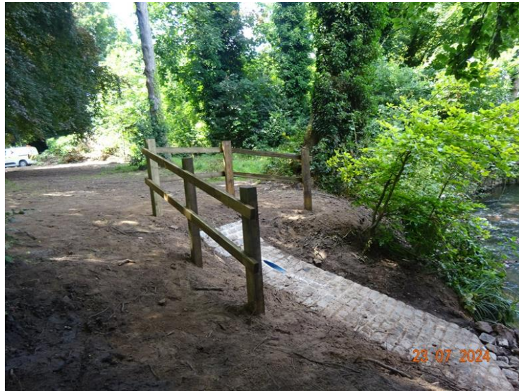
Highway Drainage Overflow System at Brookfields Park
