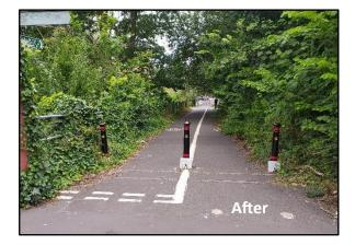
9.3 In February 2023 owing to site access for maintenance the A-frame on Lapwing Lane in Brinnington was removed. In accordance with the Access Control Policy statement, this discriminatory barrier was replaced with an accessible bollard providing a minimum gap of 1.5m.
