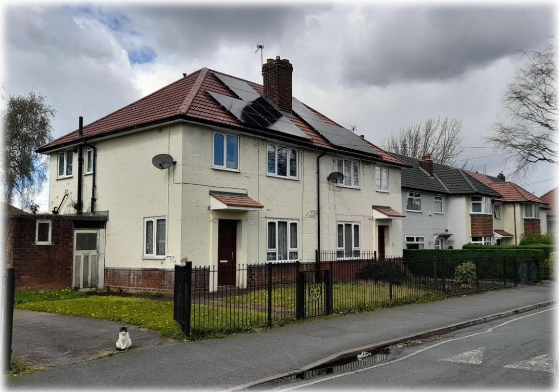
Pictures Above: New Roofing & PV on Larkhill Road, Cheadle Hulme
