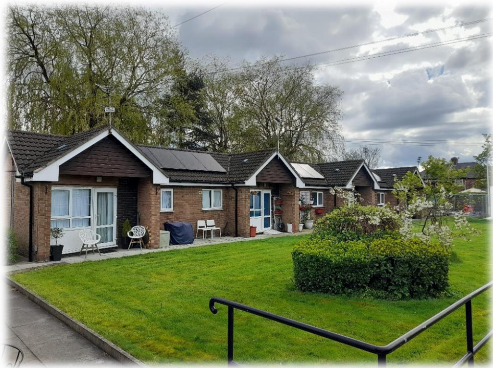
Pictures Above: New Solar Panels at Wimborne Close
