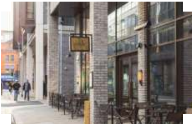
Tall and transparent ground floors and a recessed building line create space for businesses to spill-out | Ancoats, Manchester
