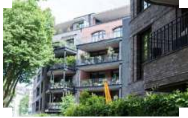
Generous windows and large balcony provision provides residents with substantial private amenity space Dusseldorf, Germany
