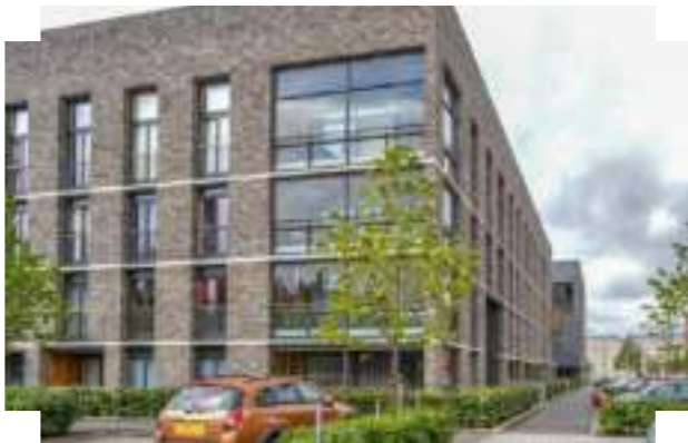
Active building frontages address on-street courtyards, permeated by green infrastructure | Laurieston, Scotland
