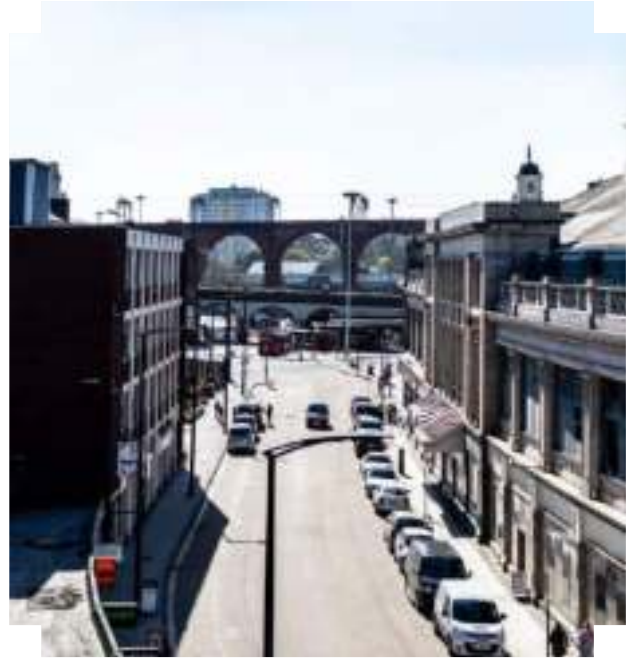
View of Stockport Viaduct from High Bank Side Bridge
