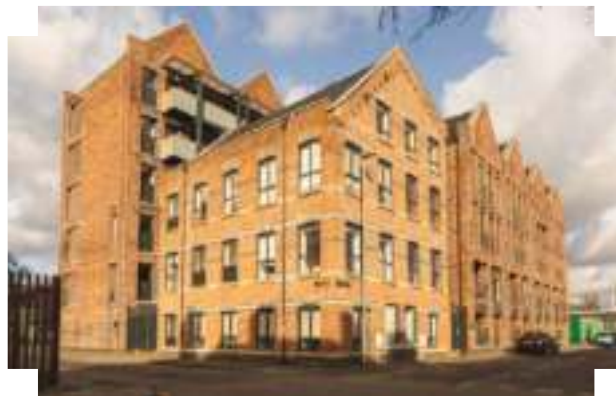
Dual-aspect apartments with habitable rooms and private amenity spaces addressing the street. The approach allows a shorter back-to-back distance and a compact urban block, without compromising residents privacy or daylight | Ancoats, Manchester
