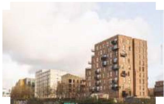
Stepping roof form and building heights mediate a transition in scale up towards the corner and key route | New Islington, Manchester
