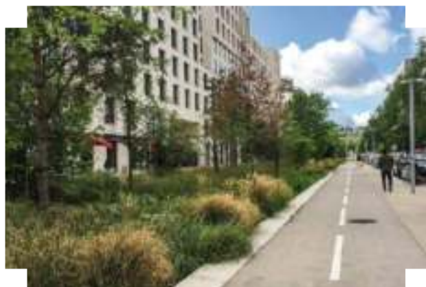
Verdant SuDS features act as a fundamental element of the street, separating transport modes and encouraging biodiversity | Parc de Billancourt, Paris
