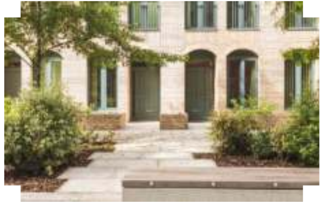
A narrow threshold, low boundary and recessed building entrance protect the privacy of residents and reinforce a fine urban grain | Embassy Gardens, London
