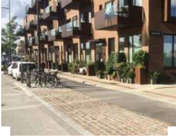
Subtle changes in complementary materials demarcate areas for different street users | Copenhagen, Denmark
