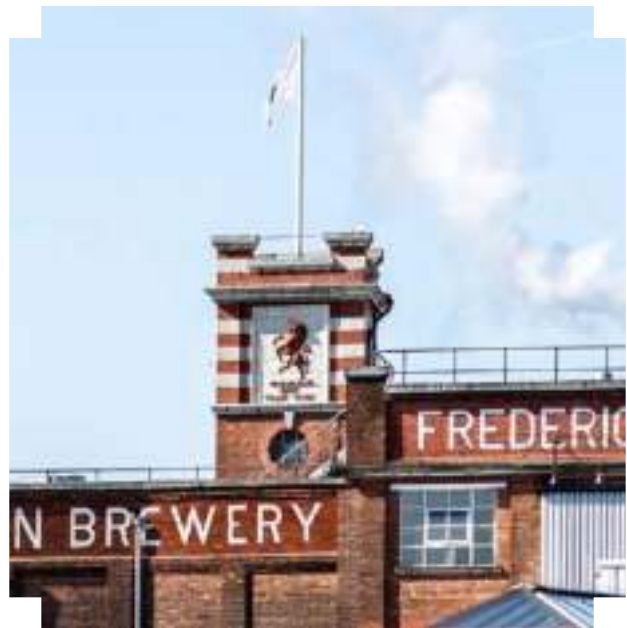
Iconic landmarks permeate the skyline across the town centre, creating markers and points of interest within the townscape | Robinson's Brewery
