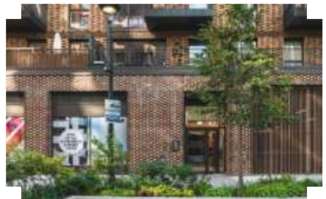
Active uses and recessed upper storeys emphasise the ground floor, contributing to human-scale at street level | Elephant Park, London
