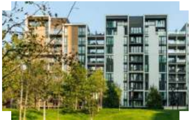
Stepping building line, heights, and recessed balconies create visual interest and depth in the elevation Victory Park, London
