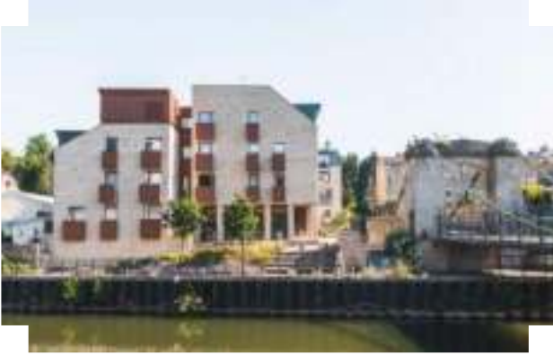
Split-level building steps up with the topography of the slope | Bath Riverside, Bath
