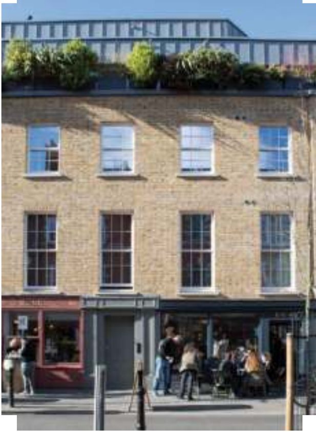
Subtly recessed upper consisting of complementary materials create raised amenity space at roof level | London
