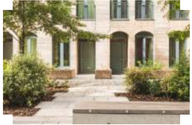
Recessed front doors and large windows address a pedestrian friendly streetscene Embassy Gardens, London
