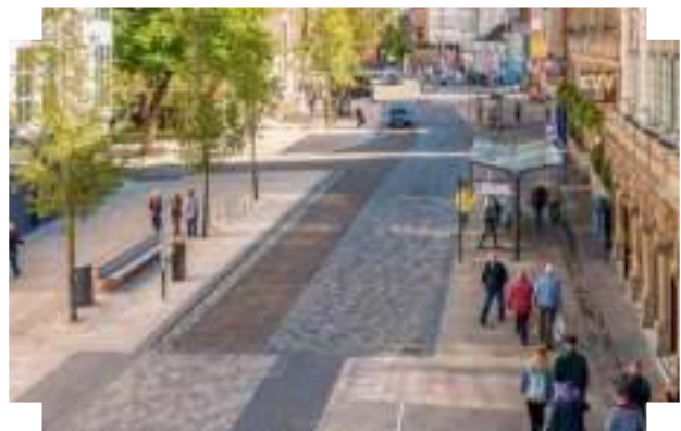
Raised carriageways and subtle changes in complementary materials contributes to a balanced streetscene. Significant carriageway space reclaimed for pedestrian activity | Fishergate, Preston
