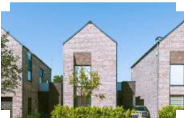
Staggered single-aspect upper storeys and narrow building footprint prevents overlooking and allows a tighter block. Private terrace integrated to the side of each home. | The Gables, Crosby
