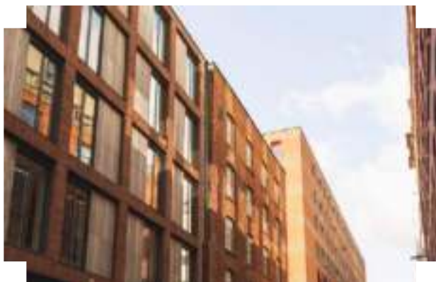
06 | A contemporary response to materiality, proportions and fenestration | Murray's Mills, Ancoats, Manchester
