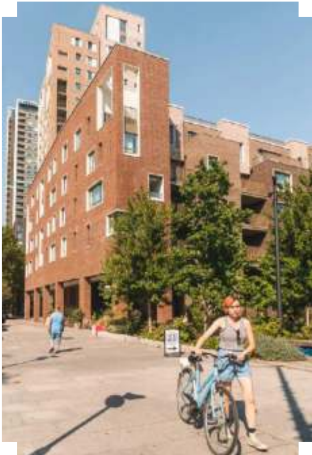
Medium-rise building heights should step up towards the corner, marking key gateways | Elephant Park, London
