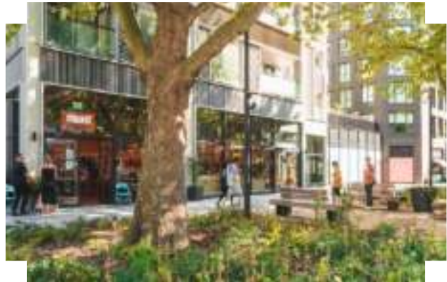
Mixed-use blocks address public realm and mature green infrastructure | Elephant Park, London
