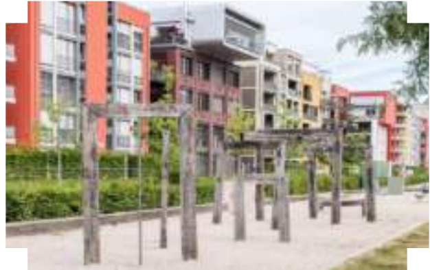
A visually interesting perimeter elevation, using mixed façade materials, accent colours, staggered building lines and stepping roof form | Dusseldorf, Germany
