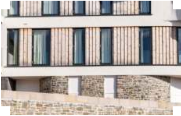
Manage value engineering to retain high-quality detailing and materials upon delivery | Bristol Harbour, Bristol
