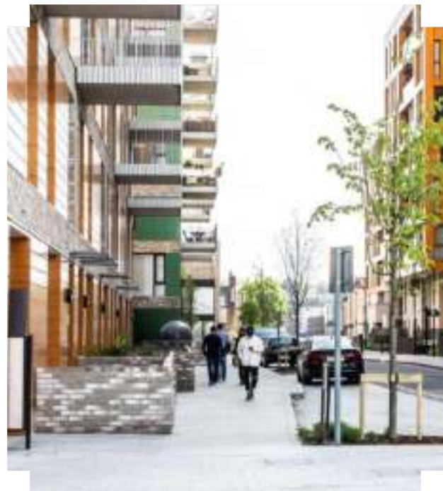
Front floors and windows address the street, with balconies raised two-storeys above street level to ensure a positive space below | Telegraph Works, London
