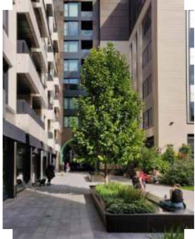
Stepping perimeter blocks lined with balconies address green streets | Rathbone Square, London
