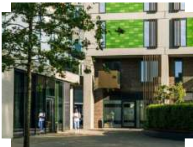
Tall and transparent entrance area creates a sense of arrival and forms a positive relationship with adjacent public space | Blackfriars, Salford
