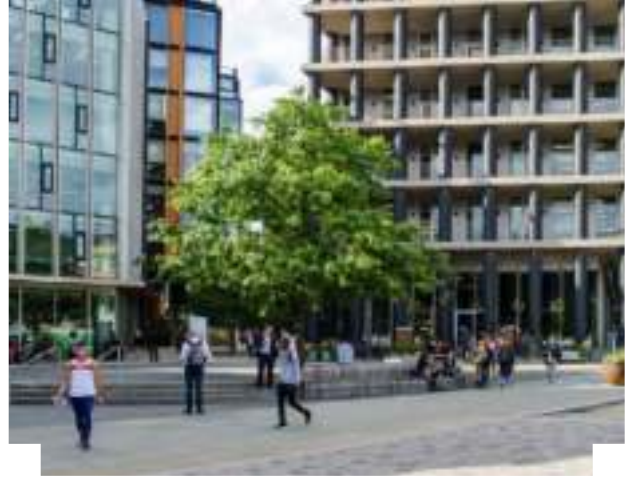
A range of mixed-use buildings create variety around a high-quality public square | Kings Cross, London
