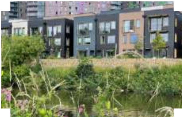
Homes adjacent to the river are raised above the river corridor using a biodiverse sloping buffer Climate Innovation District, Leeds
