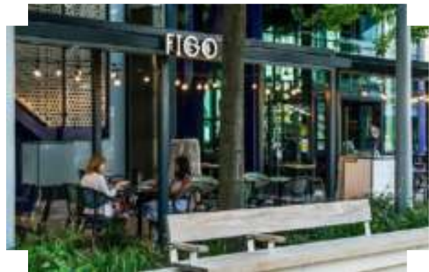
Tall, light and transparent active ground floor uses and enclosed spill-out space | Queen Elizabeth Park, London
