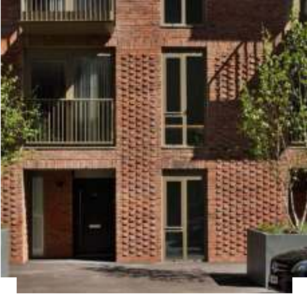
Perforated brick detailing at lower levels creates visual interest along the frontage
