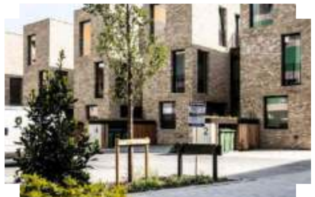
Covered and secured bin storage integrated into the curtilage of the building | Telegraph Works, Greenwich
