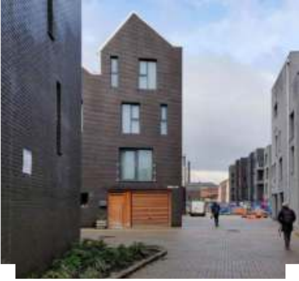
Roof form references heritage and delivers a subtle step up in height at the end of the terraced row | Little Kelham, Sheffield
