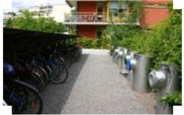
Carefully located pneumatic hatches, subtly integrated into public space | Hammarby Sjostad, Sweden
