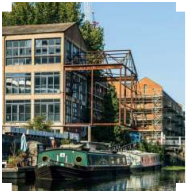
Converted industrial buildings to the rear of the image address the riverfront | London
