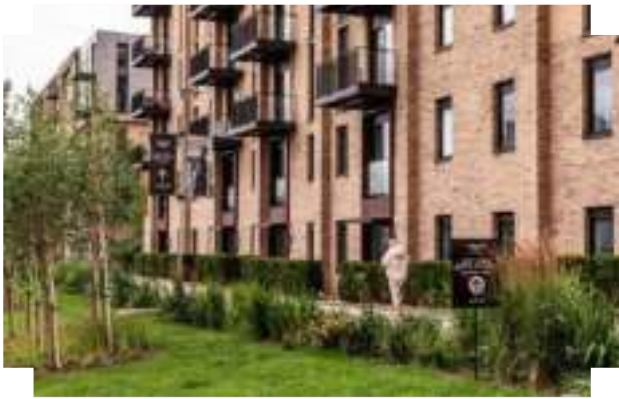
The street is structured around a central linear green and incorporates green infrastructure within the curtilage boundary | Middlewood Locks, Salford
