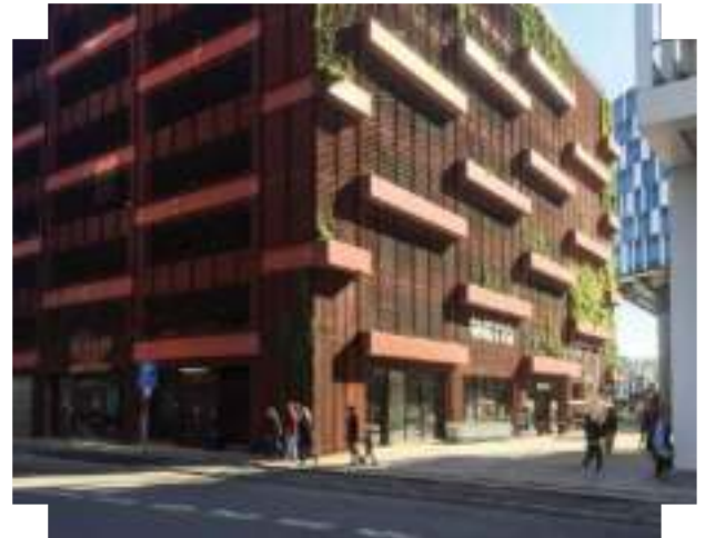
The multi-storey car park serves more than one function, with space for active land uses integrated into the ground floor and playground at roof level | Copenhagen, Denmark
