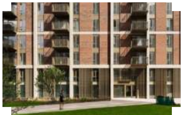
A robust set of complementary materials, detailing and vertical fenestration deliver a contemporary industrial aesthetic | The Crescent, Salford
