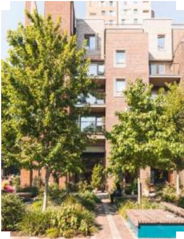
The building line is recessed at points, adding depth to the elevation and creating large inset balconies | Elephant Park, London
