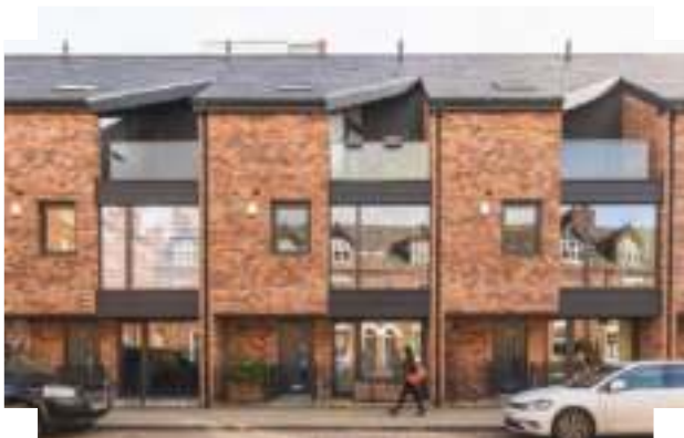
Raised amenity space at roof level and habitable rooms address the street, allowing for a more compact urban block | Ancoats, Manchester
