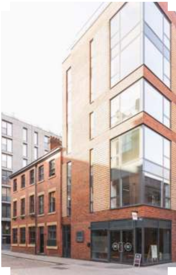
A sensitive, contemporary response to heritage which steps up to the corner | Ancoats, Manchester
