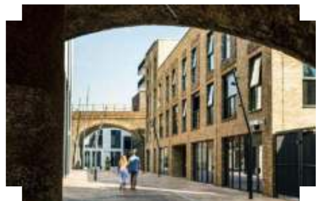
The building subtly steps up in scale to emphasise the corner | Battersea Exchange, London
