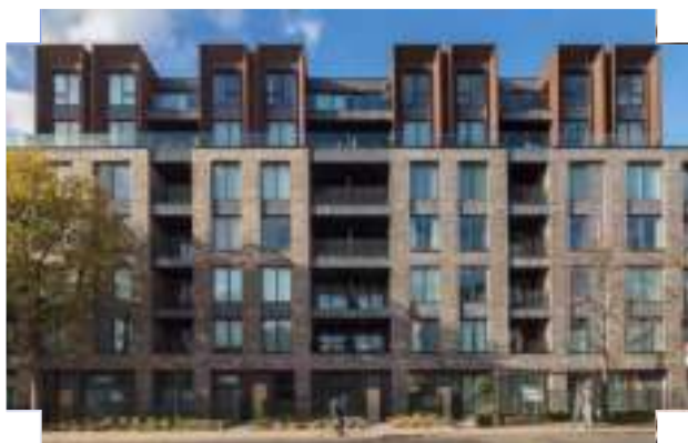
A range of complementary materials, generous windows and inset balconies create depth in the elevation | Camden Courtyards, London (Architect: Sheppard Robson / Image Source: © Simon Kennedy)
