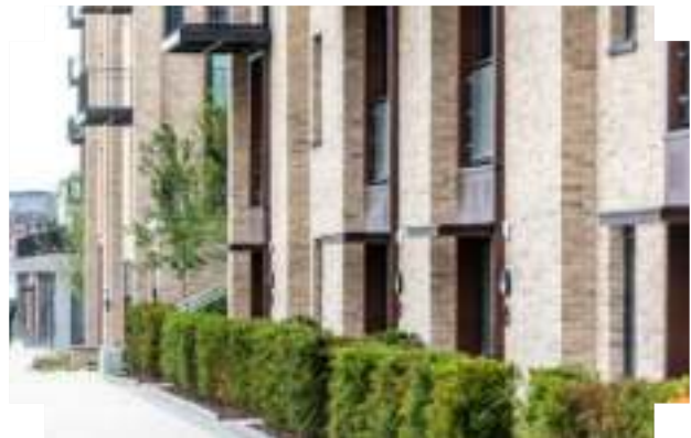
Townhouses integrated into lower floors of duplex blocks | Middlewood Locks, Salford
