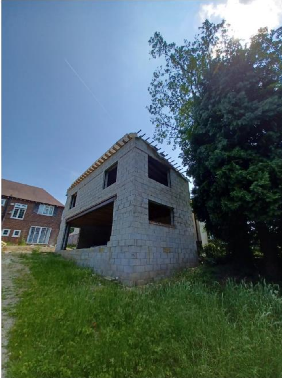
(Photo 2: Picture of Outbuilding under construction for which permission is sought)
