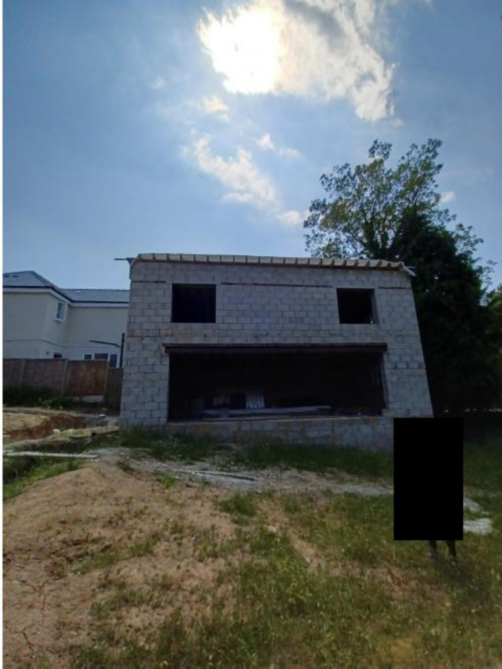
(Photo 1: Picture of Outbuilding under construction for which permission is sought)
