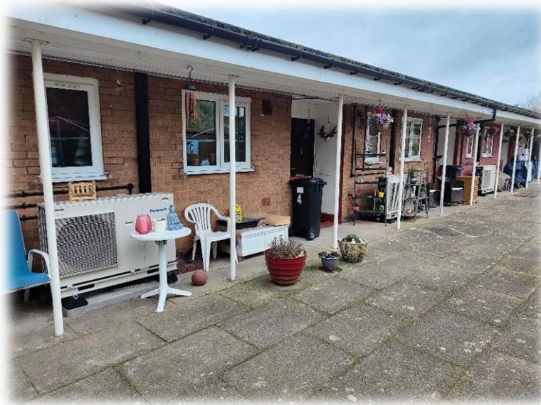
Pictures Above: (Right) Air Source Heat Pumps fitted at Garston Close (Left) New Heating Control Panel
