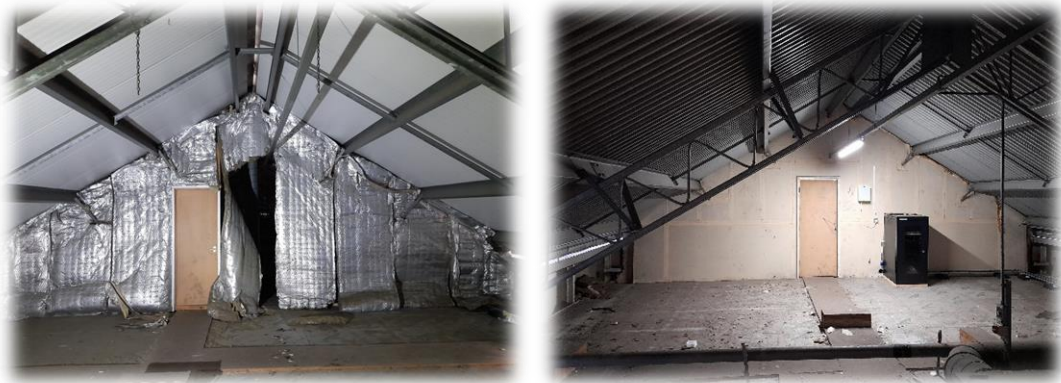
Picture Above: Dilapidated Fire barrier, before works
