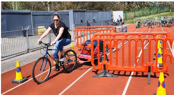
2.5m spacing of chicanes on 3m path. Picture shows bike with trailer.
