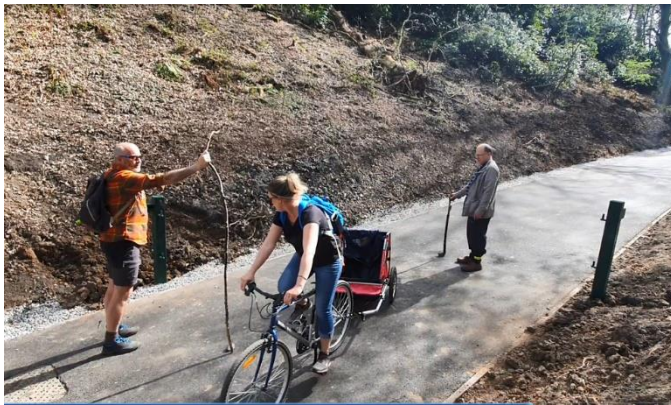
3.5m spacing of chicane on steep hill as per Sustrans guidance. Picture shows Bike With Trailer
