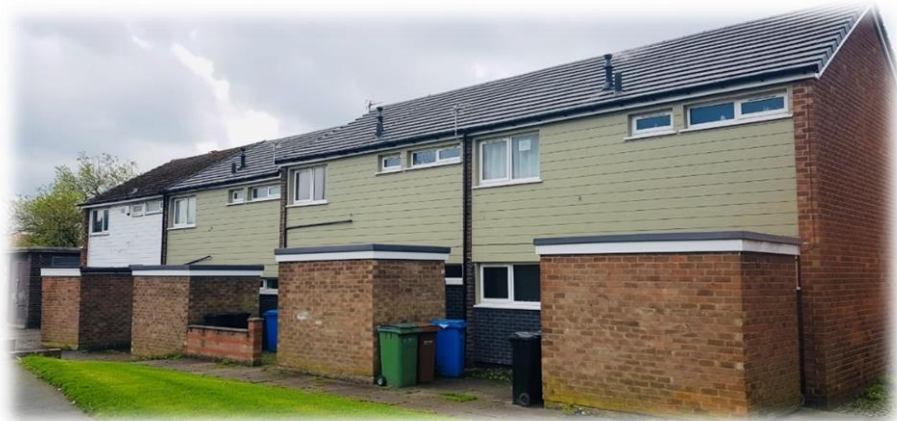
Picture Above: Examples of New Roofing, Cladding, Brick Slips, and GRP Outhouse Roofs.
