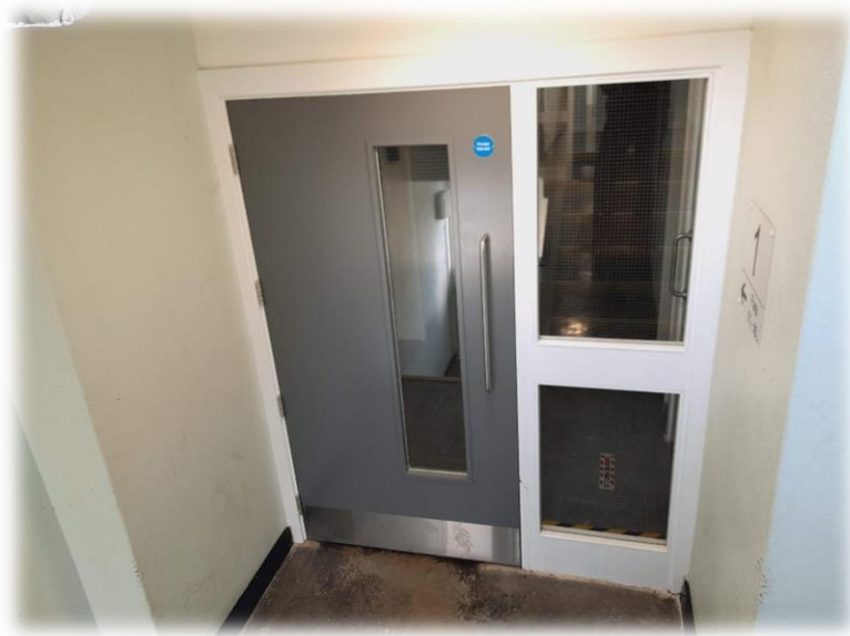
Picture Above: Examples of New Fire Rated Cross Corridor Door and Screen
