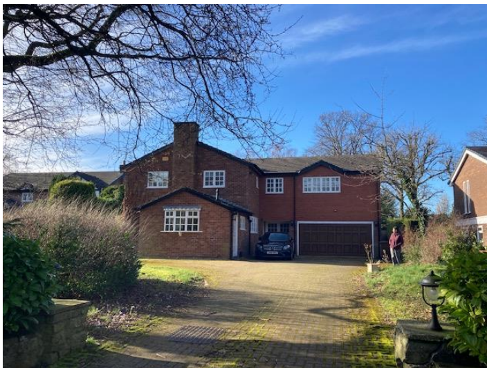
Figure 1: View of the front of Woodlands from Ladybrook Road
