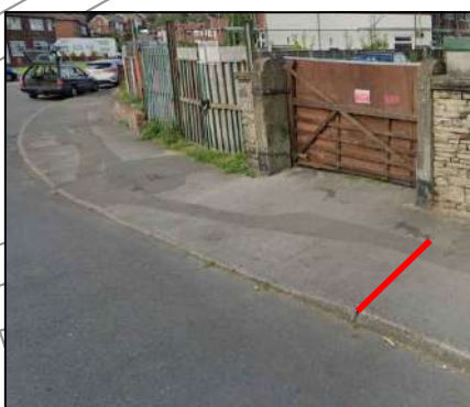
PHOTO SHOWING TRANSITION KERB AT FARM ENTRANCE
