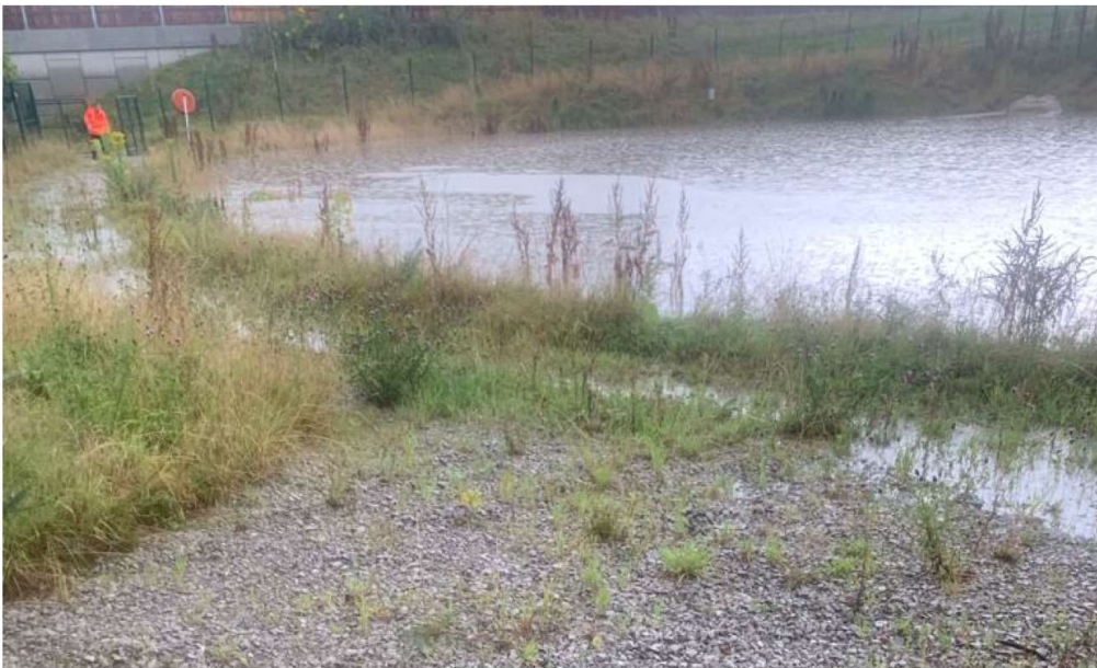
Figure 2.10: Network C attenuation pond overflowing 31 st July 2019
