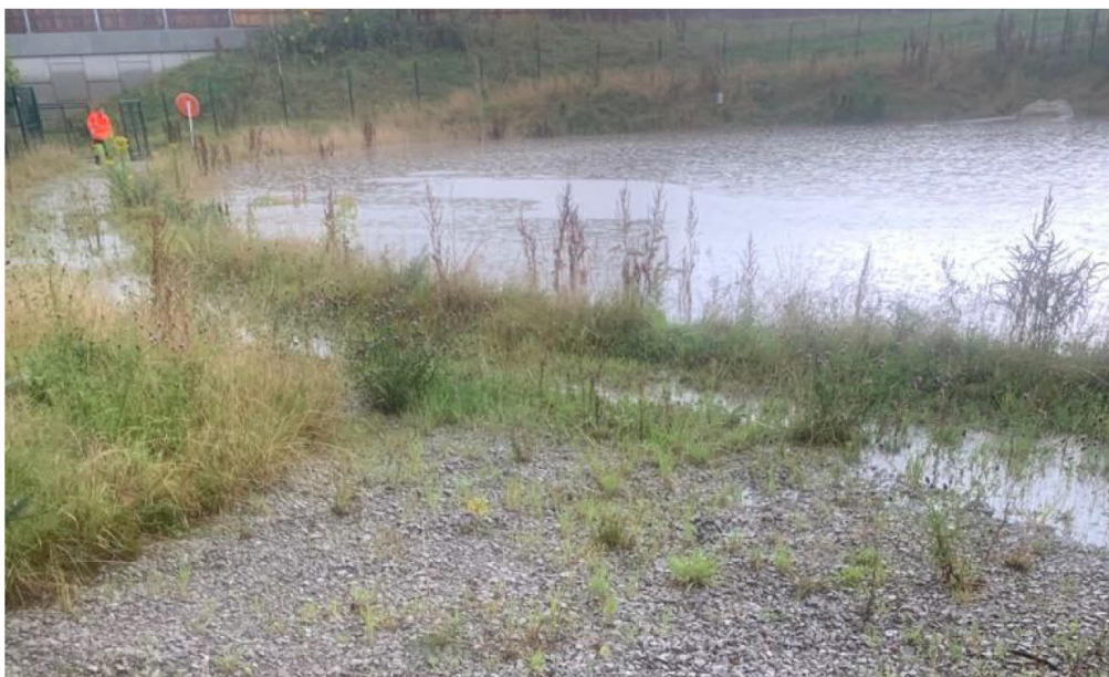
Figure B.2: Network C attenuation pond overflowing 31 st July 2019
